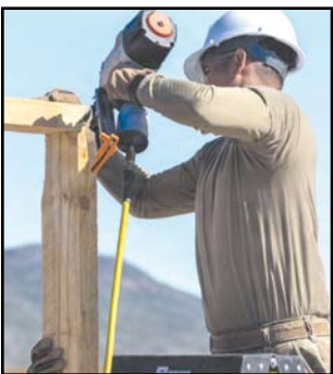
A National Guardsman constructs a new pitched roof at a lodging facility in Kangerlussuaq, Greenland, June 15. U.S. Air Force photo by Staff Sgt. Jocelyn Tuller
